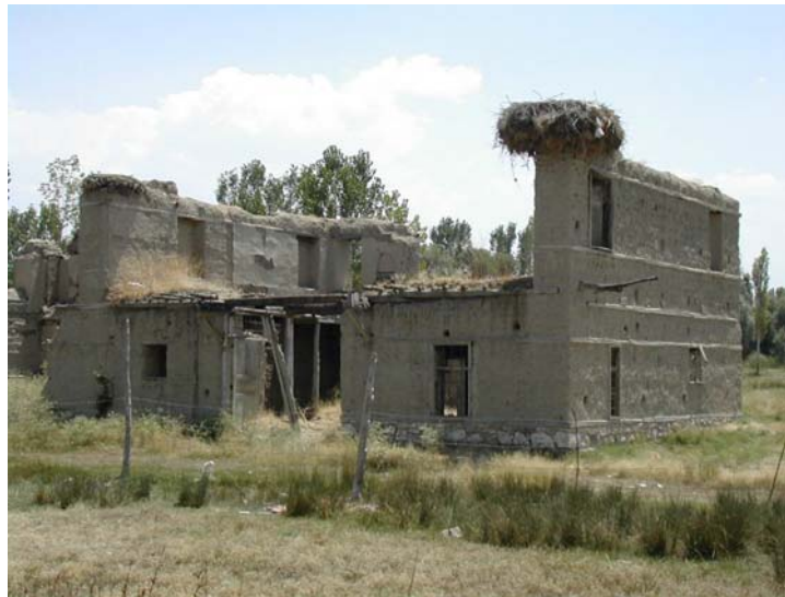
Figure 5: An abandoned house in Yazıköy: note the wooden hatıl
