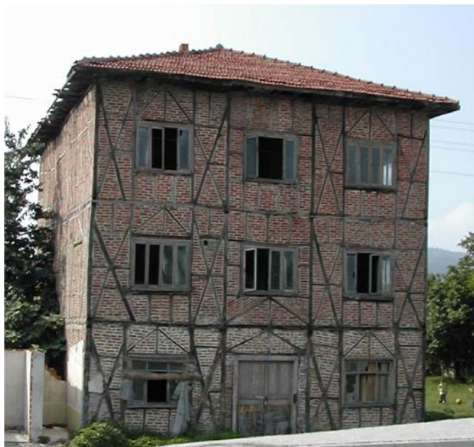
Figure 7: Traditional wood frame and brick building found along the North Anatolian Fault, Turkey.
