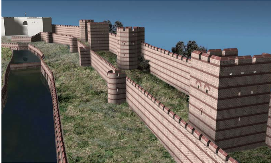
Figure 3: Computer-generated reconstruction of the land walls in Istanbul indicating the banding of the hatıl .
