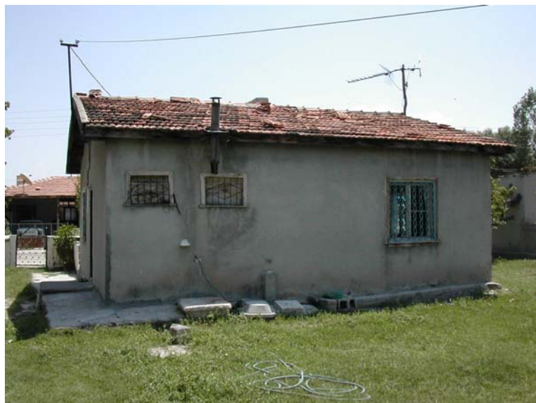
Figure 6: A government-built post-earthquake house in Yarıköy
